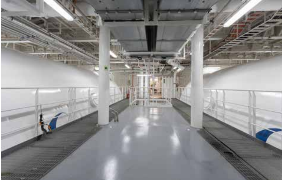
The two 400 cbm type C LNG-tanks.
