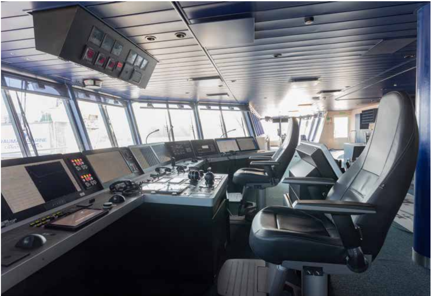
Both the bridge and the crew accommodation are located on Deck 10. Kongsberg has supplied the bridge equipment package.
