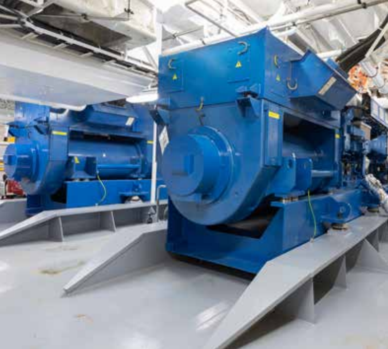
Two of the three Wärtsilä 20DF-based AUX-engines.
